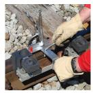
• Used to remove the slag from the crucible area of the mold after making a nVent ERICO Cadweld connection
