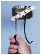
Attach SC5 bracket to inside of the box.
