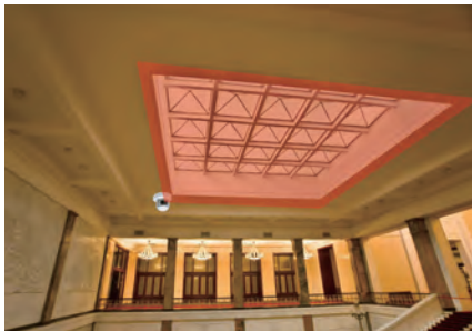
Skylight protection at Public facility / Warehouse
