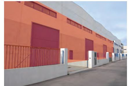
Wall protection (outdoor) at Warehouse
