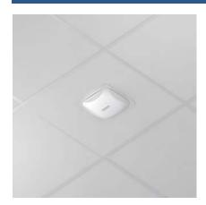
Model 1040 is an economical, easy-to-install cloud or canopy mounting kit for WAPs from most vendors. A cutout is made in the ceiling panel, the panel bridge is placed above the ceiling panel, and the white trim is placed around the WAP. The WAP is attached to a universal mounting T-bar and pressed into the panel bridge. The WAP is now recessed into the ceiling much like a recessed light fixture for unobstructed wireless coverage. WAP trim can be swapped out for alternate WAP brands.
