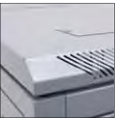
Multiple roof access points
