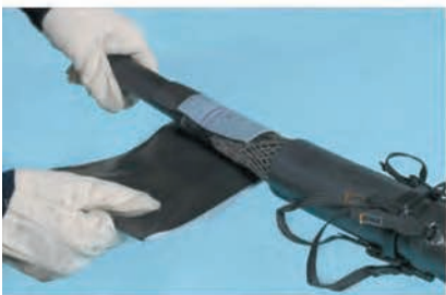
Applying sealing mastic
