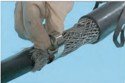
Connecting the shield braid to the cable metallic shield
