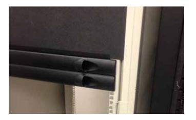
5. Repeat the process to enclose the openings on the rack. The sizes and Blanking Panels can be used interchangeably in any configuration.
