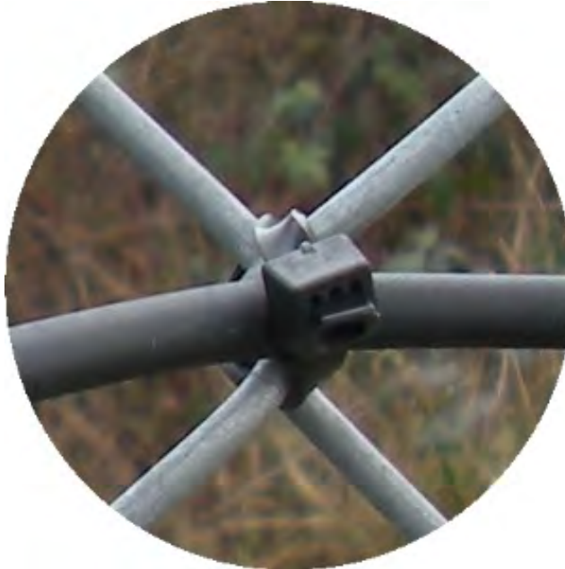
Figure 4-2. Correctly tied through vertically adjacent diamonds.
