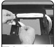
A Route cable onto tray and fasten with hook and loop managers. Tray allows routing of cable along three separate horizontal pathways via three rows of hook and loop managers. Cable bundles can then be routed down the middle and/or sides of tray (as shown).
