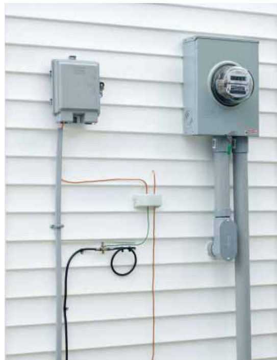
Intersystem Bonding Termination - Typical installation bonding the electrical system to the telephone and CATV systems.
