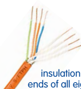
Open the four twisted wire pairs
