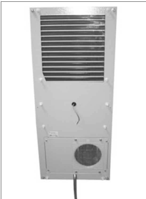
Fig. 47: Cooling unit without grille
