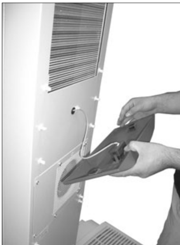
Fig. 66: Remove the infill panel
