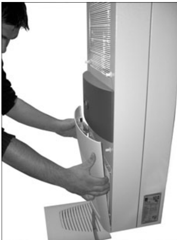
Fig. 43: Remove the lower louvred grille
