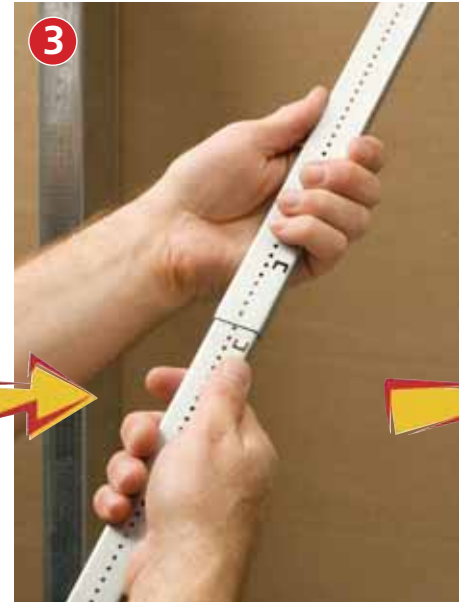
3. Slide one arm on top of the other until you hear a click.
