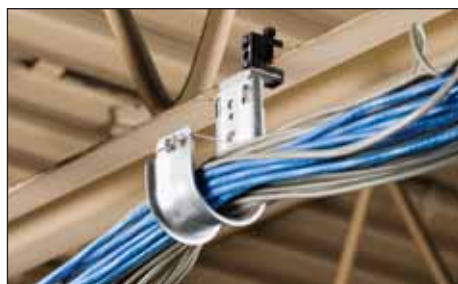
CATHPBCB for 1/8" – 1/2" flange with 360° rotation
