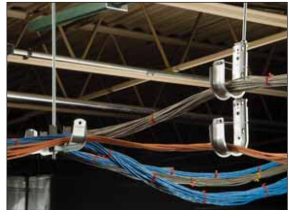
CADDY® CAT LINKS branching off from a CADDY® CAT CM
