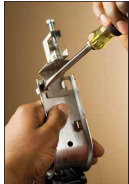
Step 3: Using a screwdriver, bend the Locking Tabs to firmly secure the J-Hook Assembly
