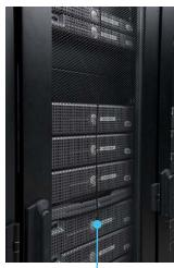
Rack sensors ensure the correct amount of cold air is provided to eliminate hot spots.
