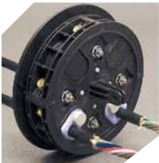
Install remaining cables and end plates caps
