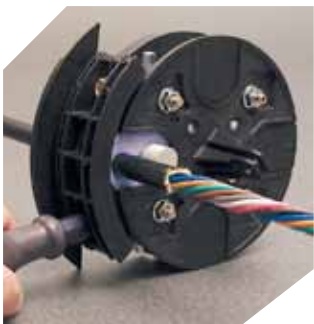
Install first of the segmented end plates caps over cable
