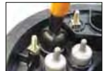
Field Installation of Hardened Adapter
