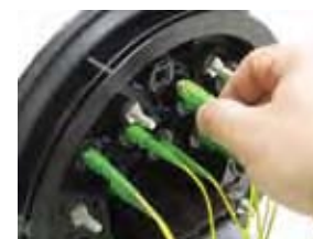
Installing Pigtail Connections
