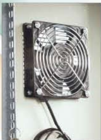
Side panel installation
