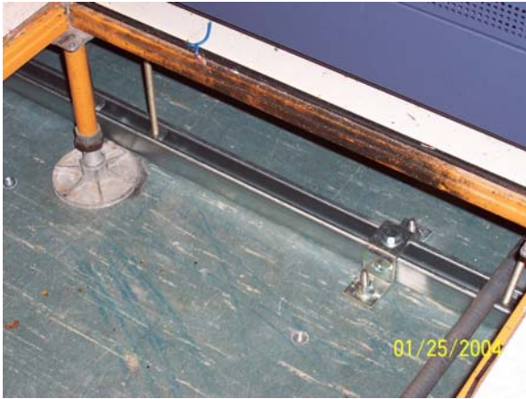
Fig. 2.2.1 Subfloor bracing
